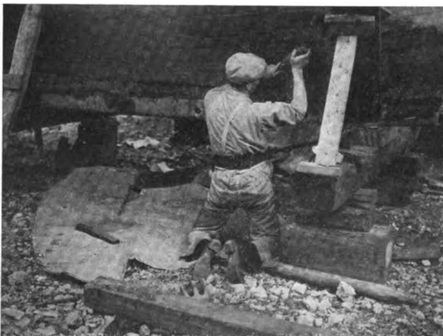
Cleaning Off the Bottom with a Wire Brush
